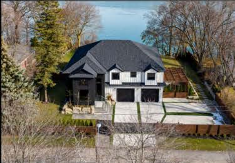
14621 NIAGARA RIVER PKWY NOTL
