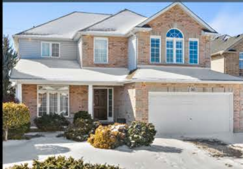
365 HILLSDALE RD WELLAND
