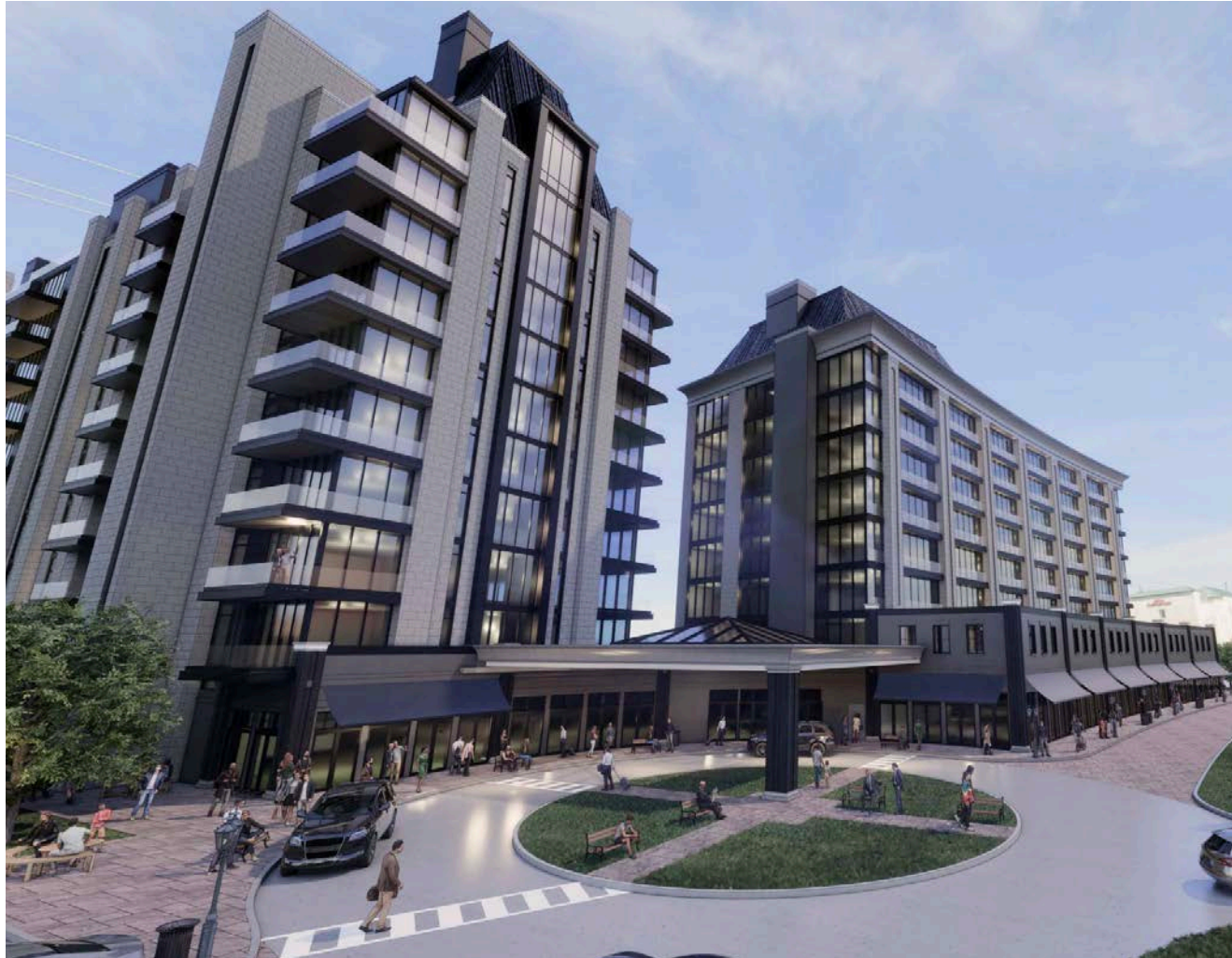
Columnist Brian Marshall says the proposed Mavridis hotel and condominiums in Glendale is a great application, though it still requires design refinement to serve as a part of Niagara-on-the-Lake's gateway. SOURCED
