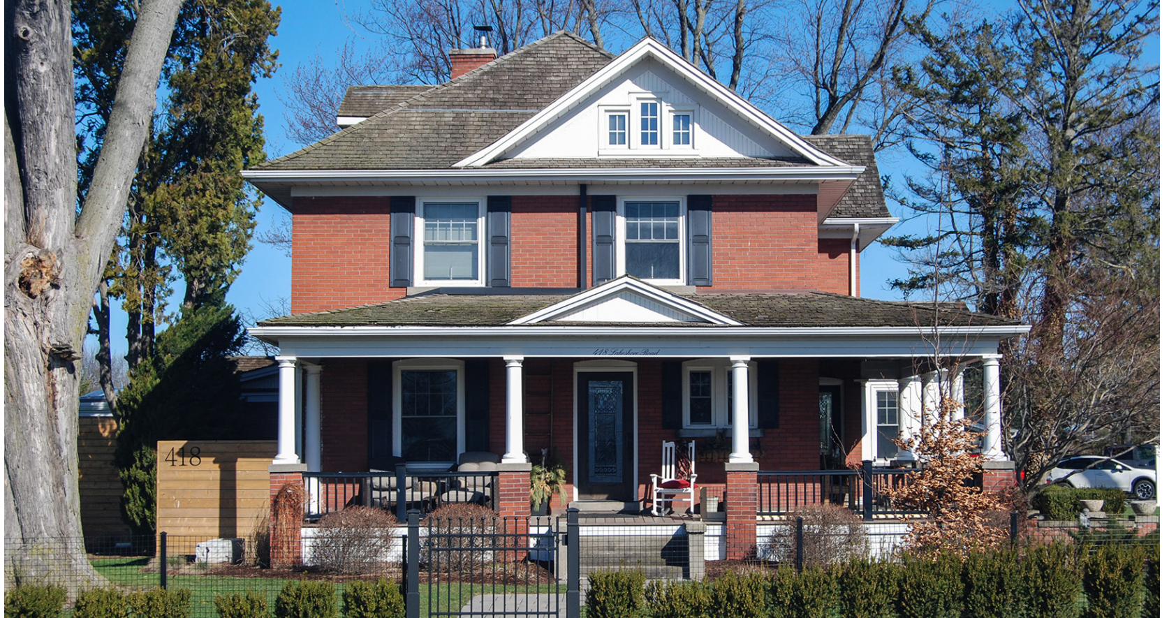
Columnist Brian Marshall says this home at 418 Lakeshore Rd. is one of NOTL's fine examples of Canadian Edwardian Classicism. BRIAN MARSHALL
