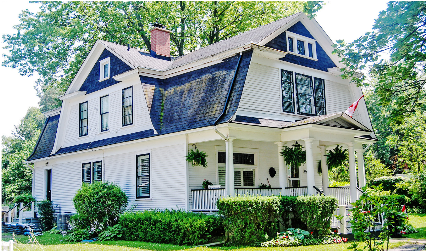
McClelland House at 164 Victoria St. is a unique and scholarly cited example of one of NOTL's Eclectic Dutch Colonial Revival homes. BRIAN MARSHALL
