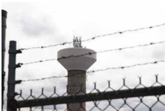
Some provincial electricity changes won’t affect NOTL customers much, says NOTL Hydro president Tim Curtis. DARIYA BAIGUZHIEVA
