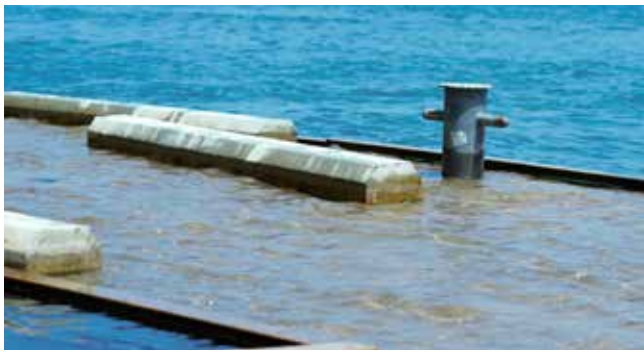
Flooding at the Navy Hall dock in 2019. FILE/BRITTANY CARTER
