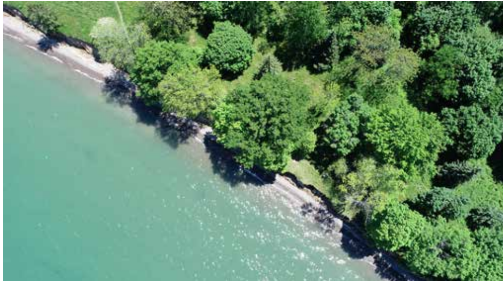
A photo of the erosion at Niagara Shores Park taken in July 2019. Since then most of the trees at the edge of the row have fallen into the lake. RENE BERTSCHI Watch The Lake Report's documentary on erosion and see past coverage at www.niagarashores.com .
