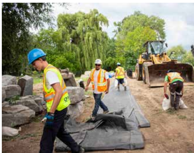
Workers building the groyne in August 2020. FILE PHOTO
