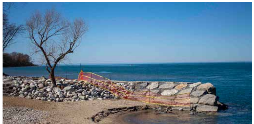
A newly built rock groyne at Balls Beach collapsed months after being built. Now the town is seeking answers about why the $400,000 project failed. FILE/RICHARD HARLEY
