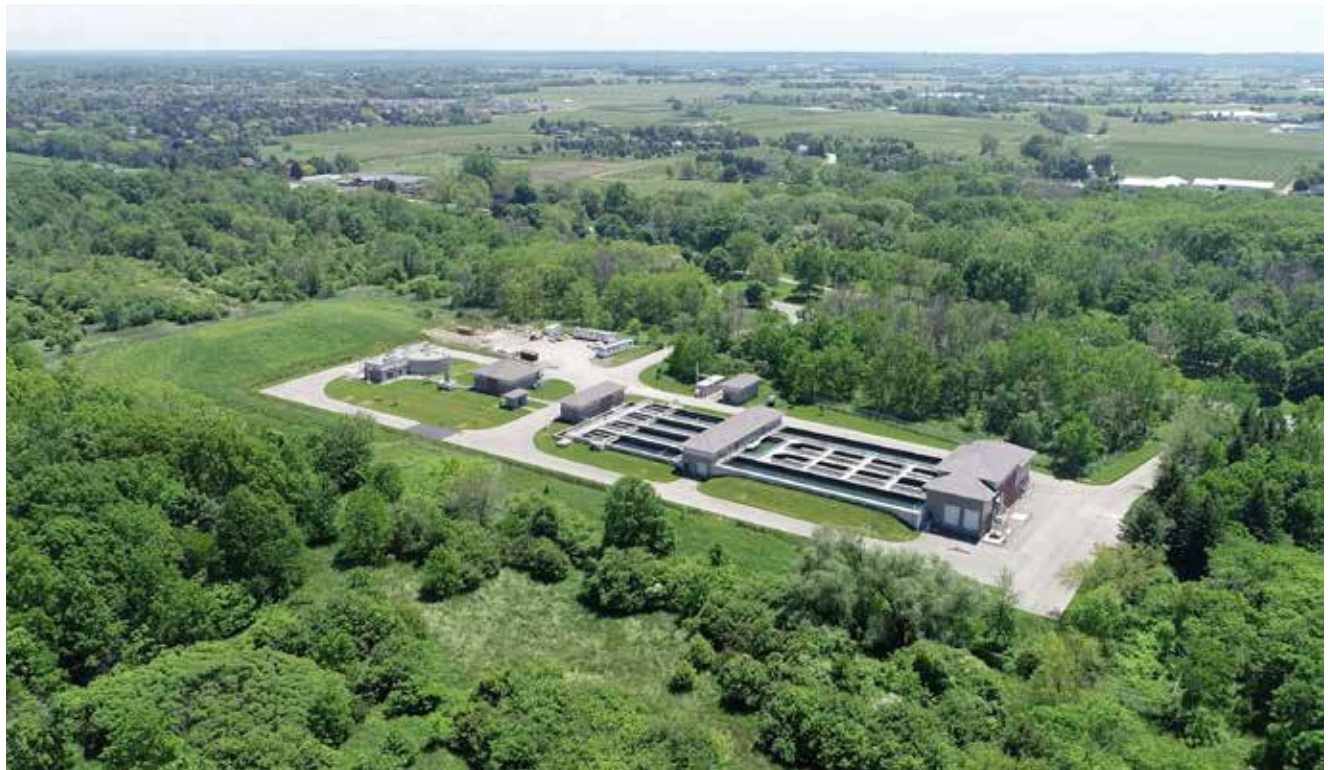
Aerial photo of the new NOTL sewage treatment plant. RENE BERTSCHI
