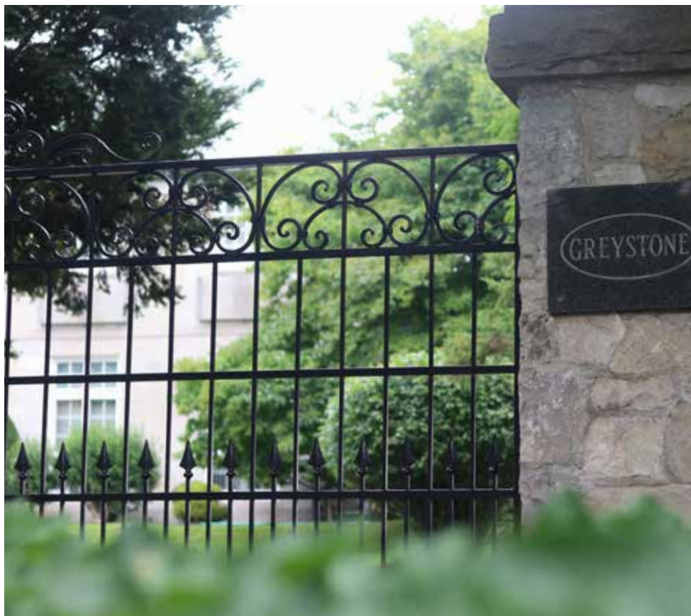
The exterior stone of the Greystone house is made from limestone from the Queenston Quarry. DARIYA BAIGUZHIEVA
