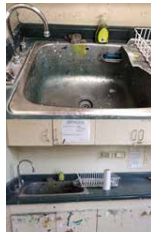
A Pumphouse sink before renovations. SUPPLIED
