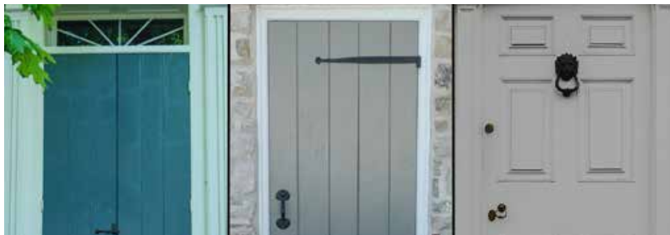
Pictured from left, storm door shutters, a double plank door and six-panel door. BRIAN MARSHALL
