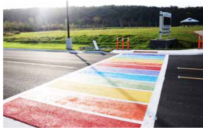
Niagara College managed to install a rainbow crosswalk in one day in 2019. FILE PHOTO
