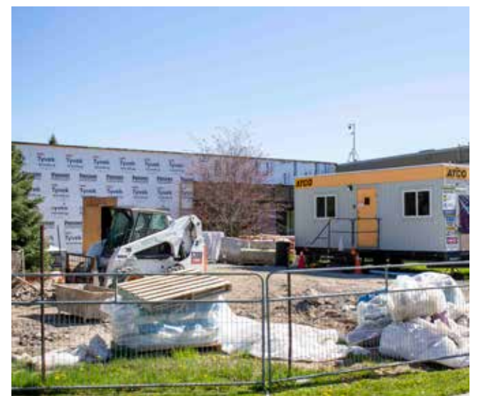
Construction on the new nursery school expansion. EVAN SAUNDERS
