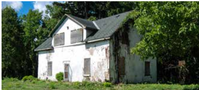
Secord-Paxton House crumbling away. BRIAN MARSHALL
