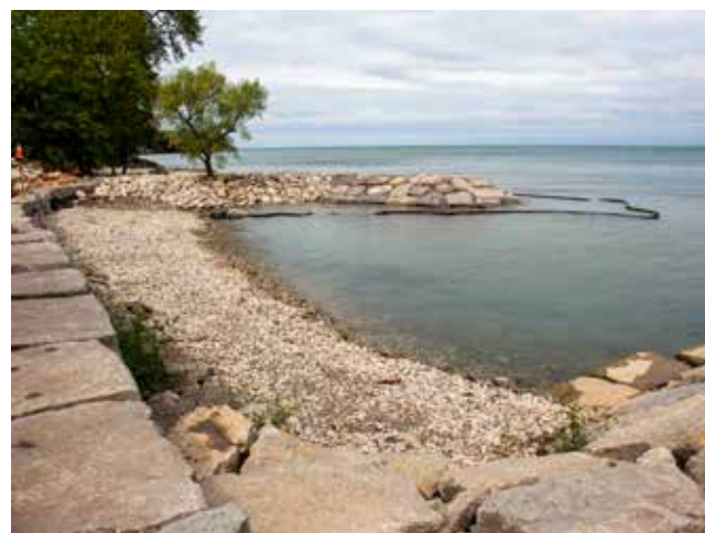
The newly renovated Ball's Beach. FILE PHOTO
