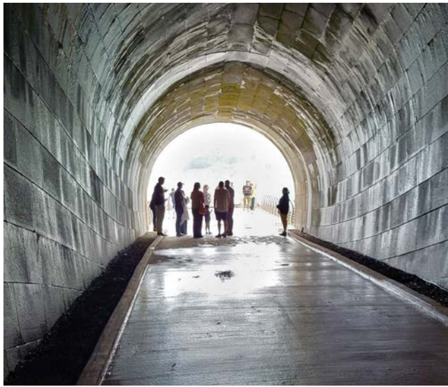
The recently opened Niagara Parks Tunnel. SUPPLIED
