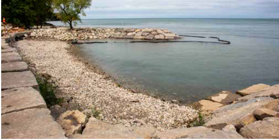
Ball's Beach after shoreline protection work this year. RICHARD HARLEY
