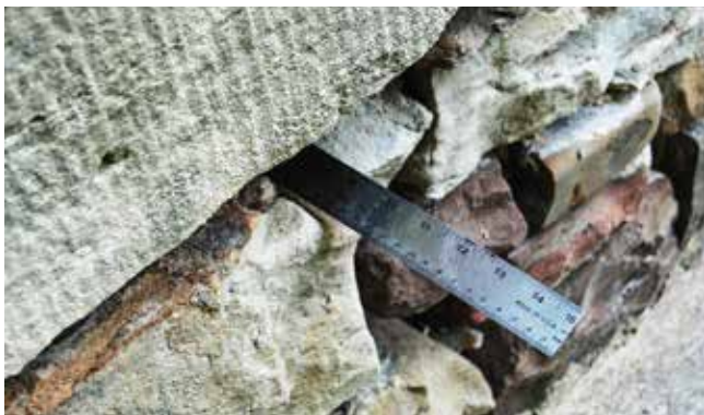
Mortar Loss hidden by Pebbledash Parging. SUPPLIED
