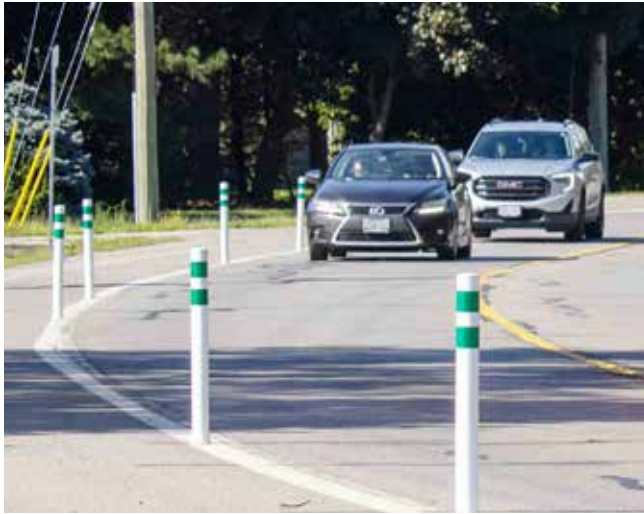
Region workers had to park on private property to install these bollards to prevent people from parking. SUPPLIED
