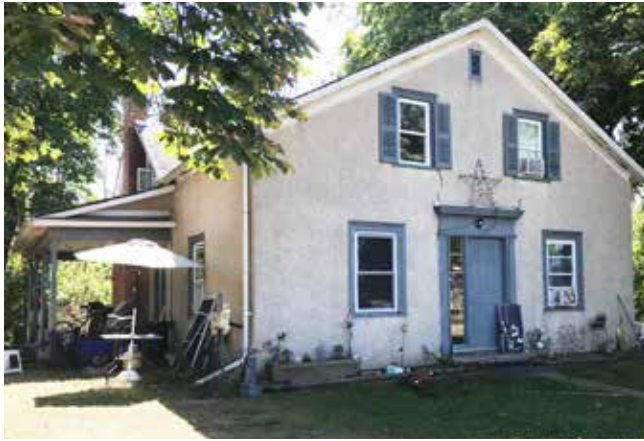
The Gordon Hunter-Dick house is one of the oldest buildings in Virgil, originally built in 1796 by John Young. DAVID HEMMING
