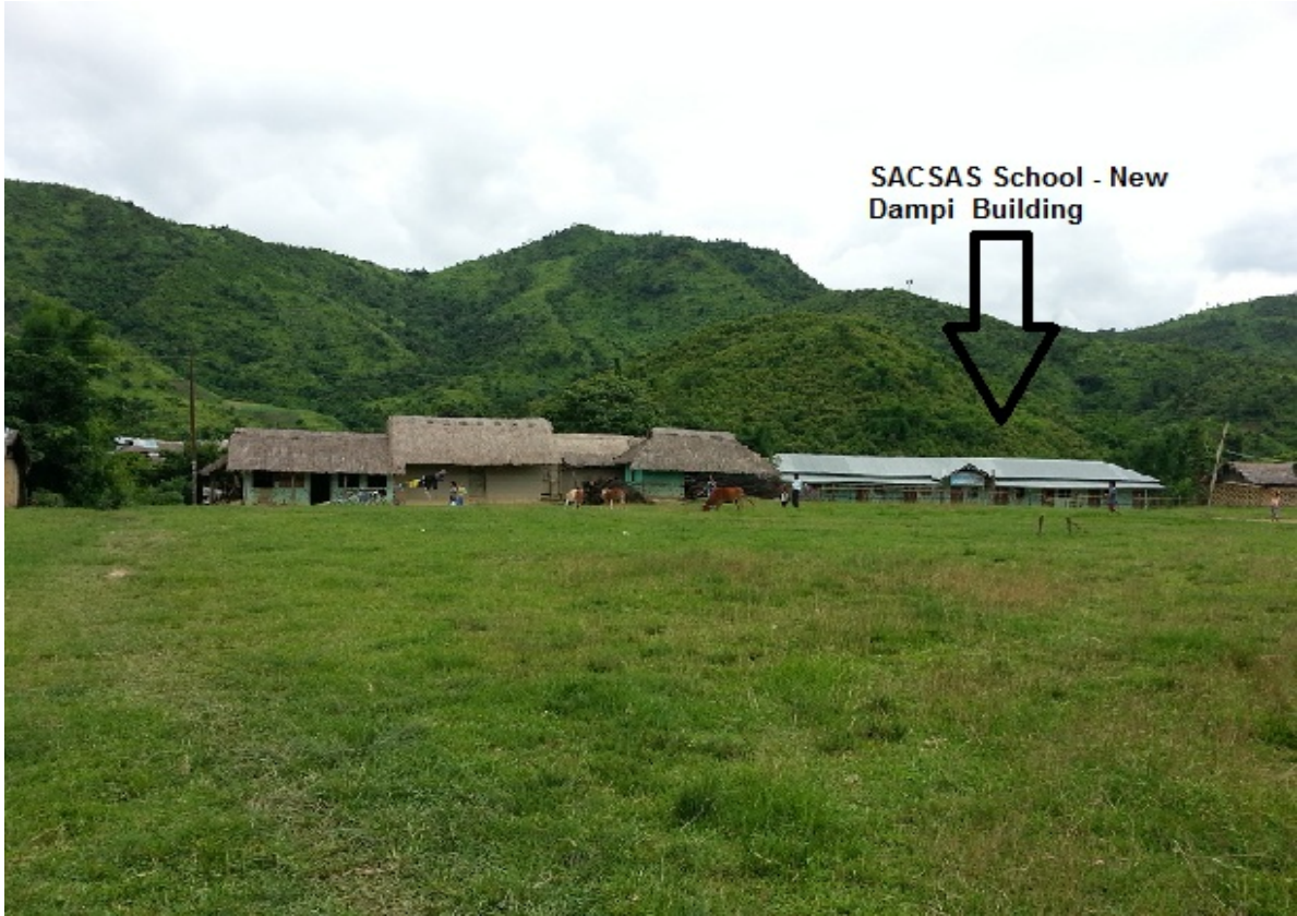
(New Dampi School Building from a distance)
