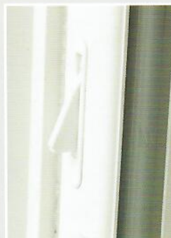
Sash vents limit the opening of the bottom sash.
