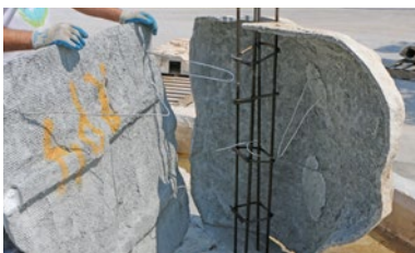
1. Columns are clam shell pieces wired to a rebar column.
