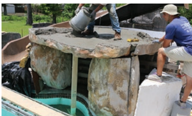
4. Top requires 1 yard of concrete. Note T brace under front grotto.
