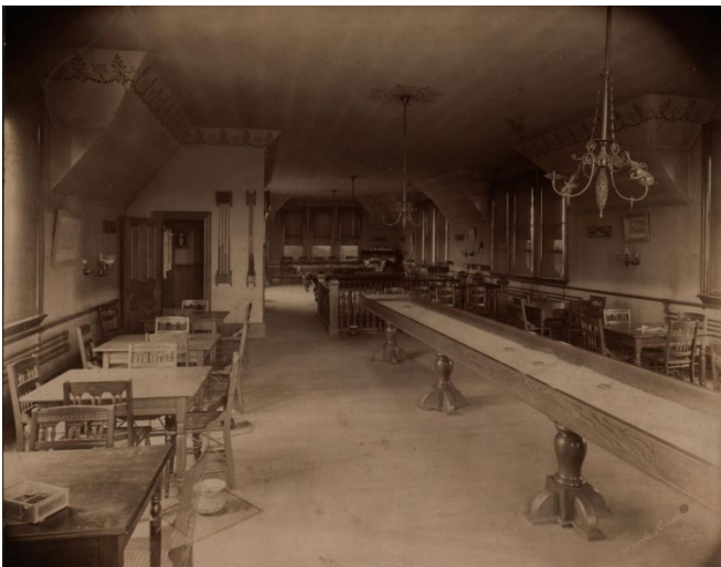
Third Floor - looking west Circa 1900
