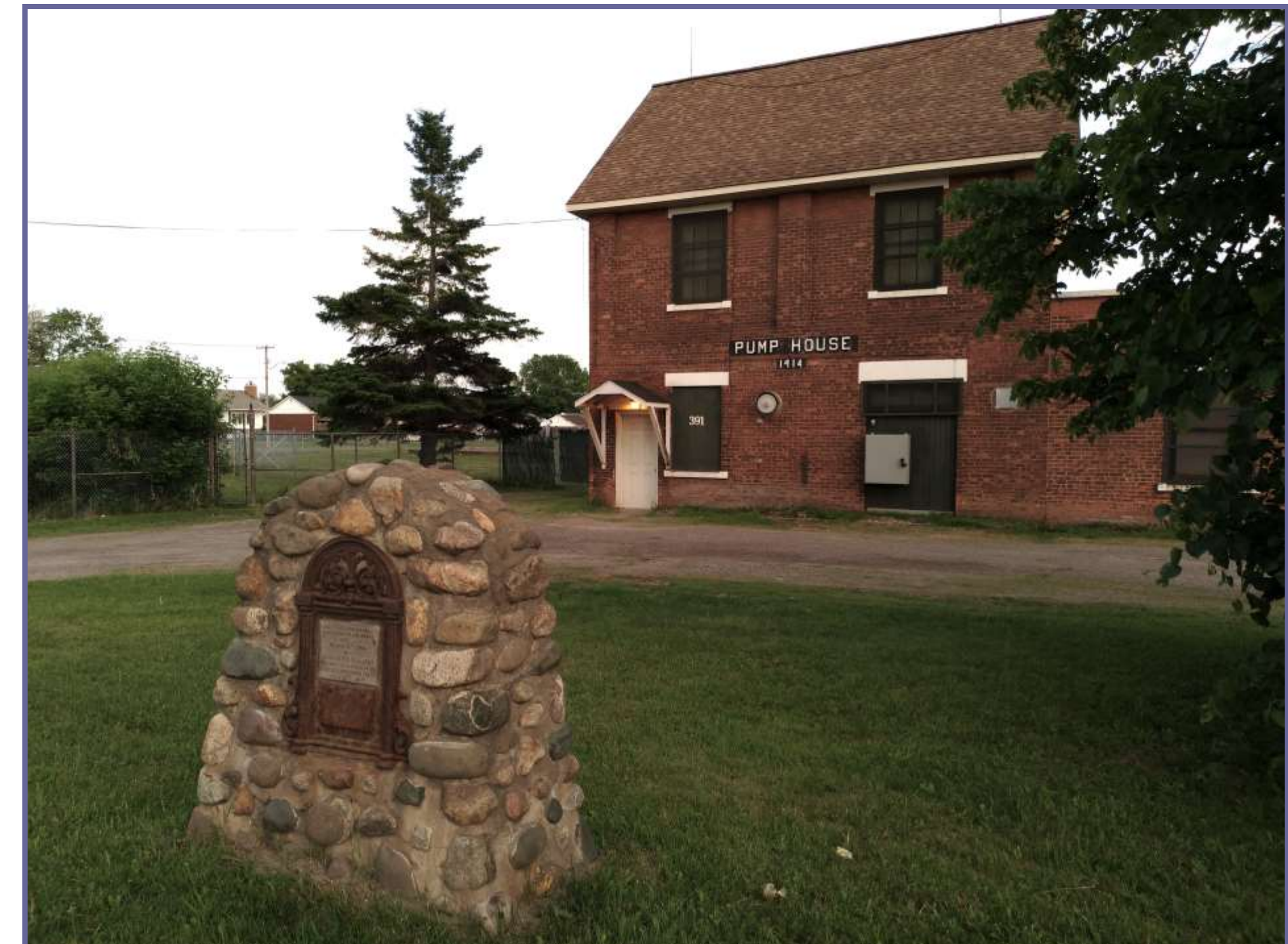
The historic "Steelton wells" pump house on Second Line West near Korah Road.
