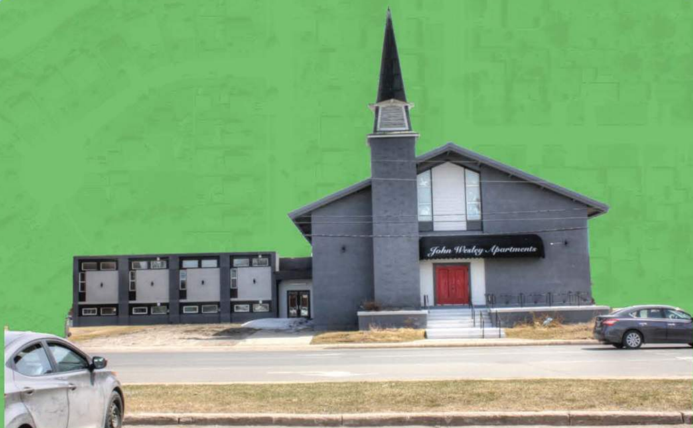
A former church was converted into a multi-unit dwelling.
