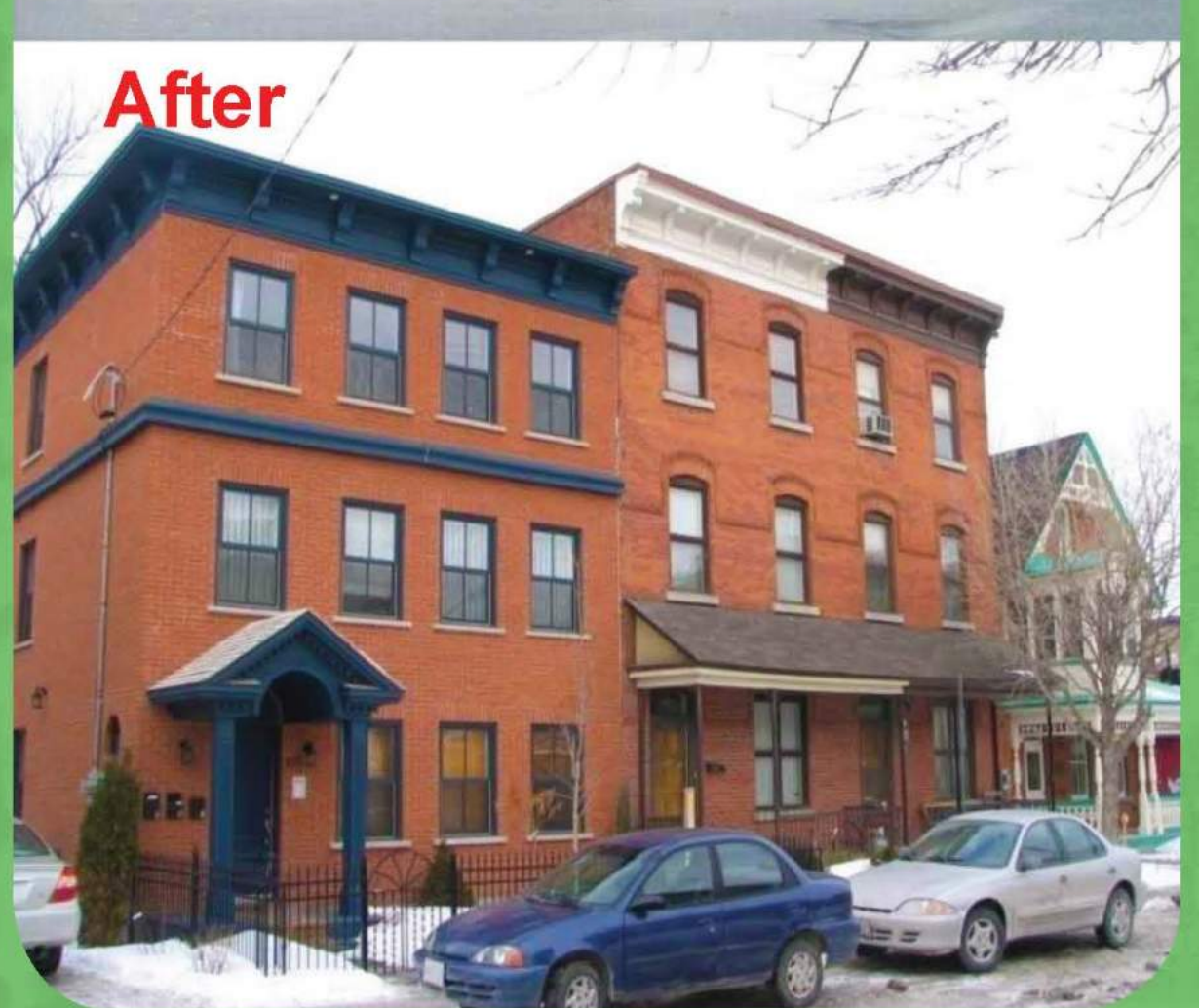
The small house on the left was replaced with a condominium. This is an example of a redevelopment of an underdeveloped lot.
