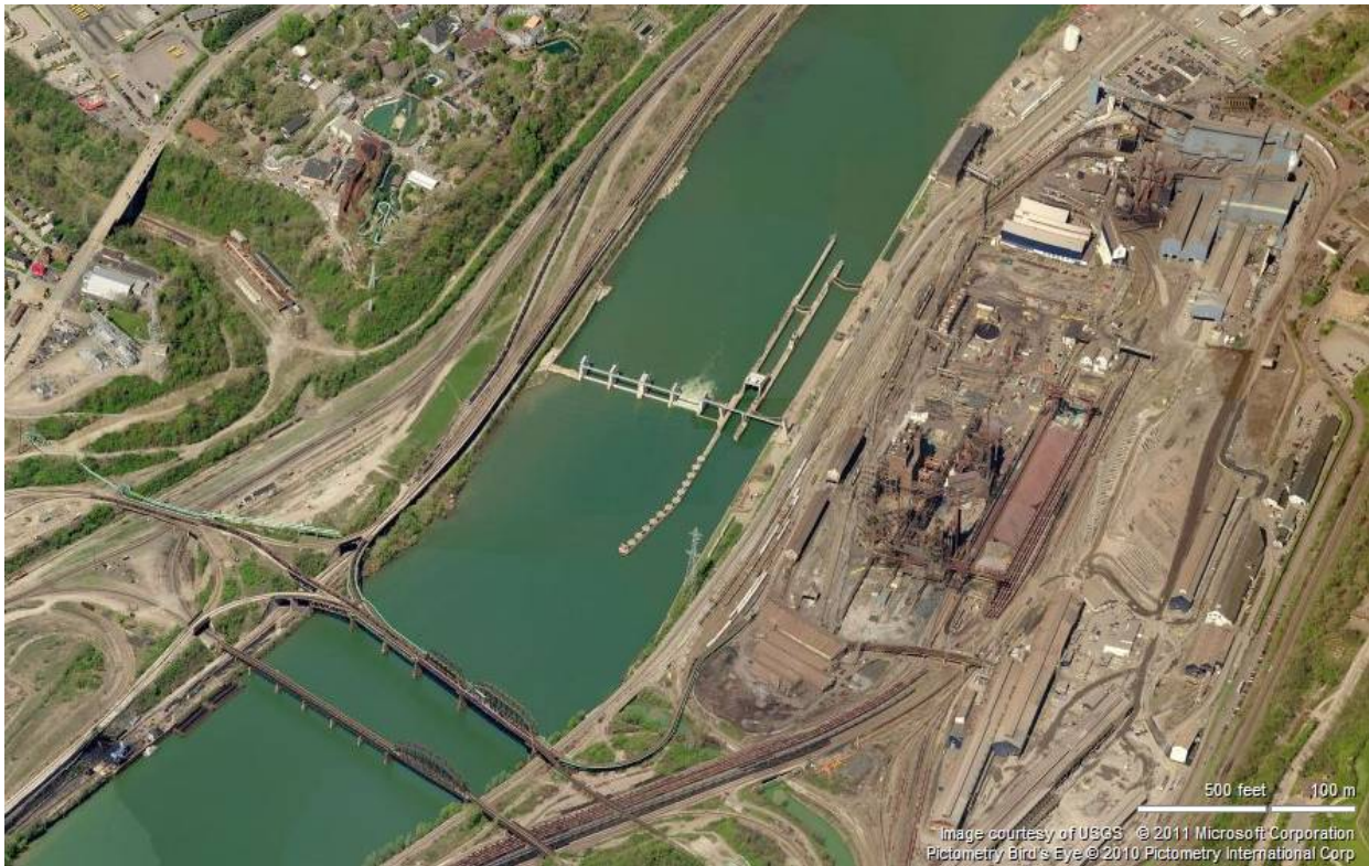
Figure E.9.1-2 Upstream aerial view of the Braddock Locks and Dam and surrounding vicinity.
