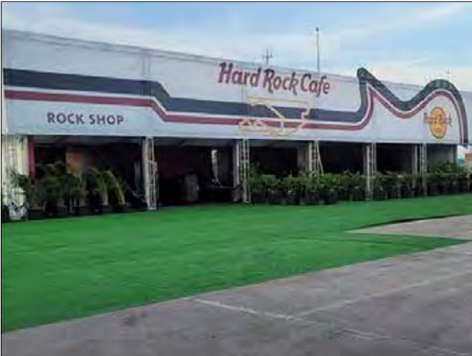
Miami Stadium Cafe and Rock Shop for F1 (temporary) Photo by Tom Krüger
