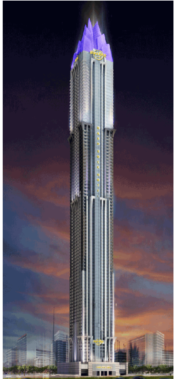
Dubai (project cancelled)
