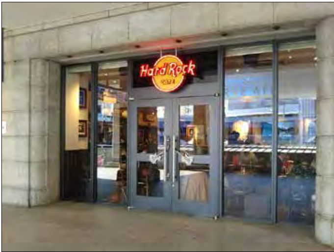
Tokyo Ueno-Eki Station Street Level
