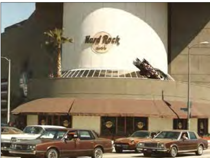
Los Angeles (original facade)
