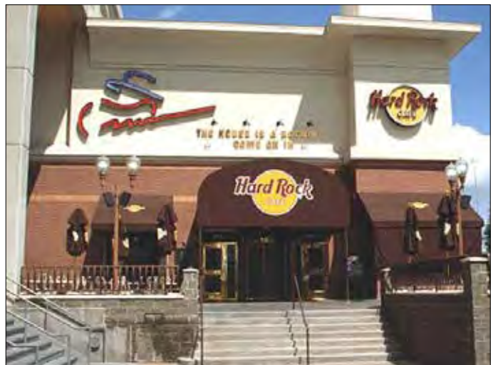
Houston (entrance with new facade)
