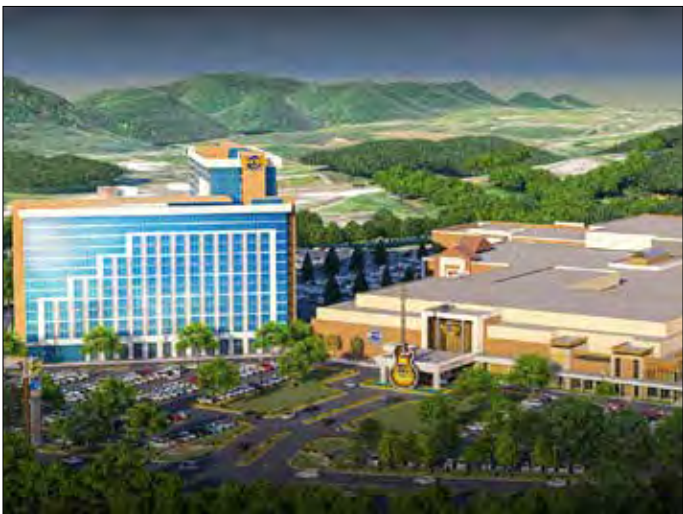
Bristol Hotel and Casino (opening 2024)
