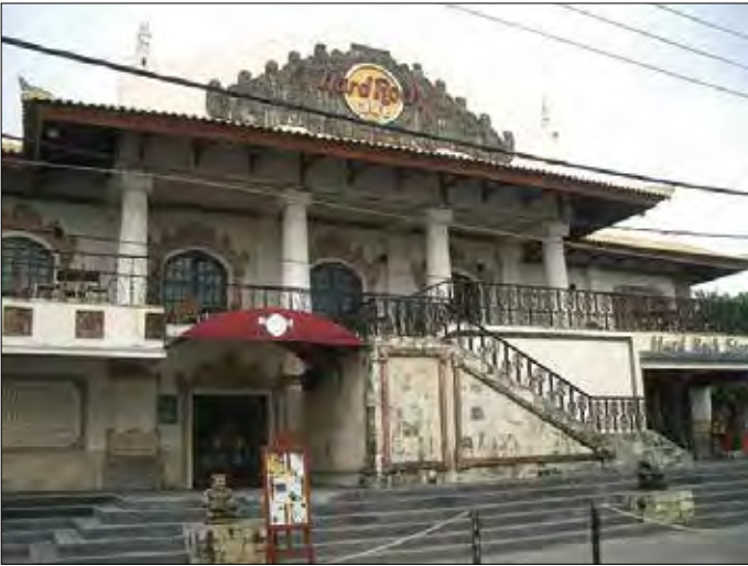
Bali (before renovation)
