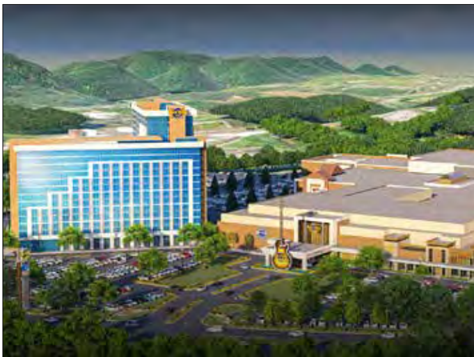
Bristol Hotel and Casino (opening 2023)
