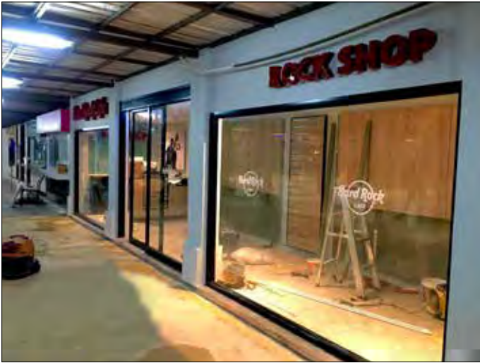
Koh Samui Airport (under construction) Photo by Kay Kalkbrenner
