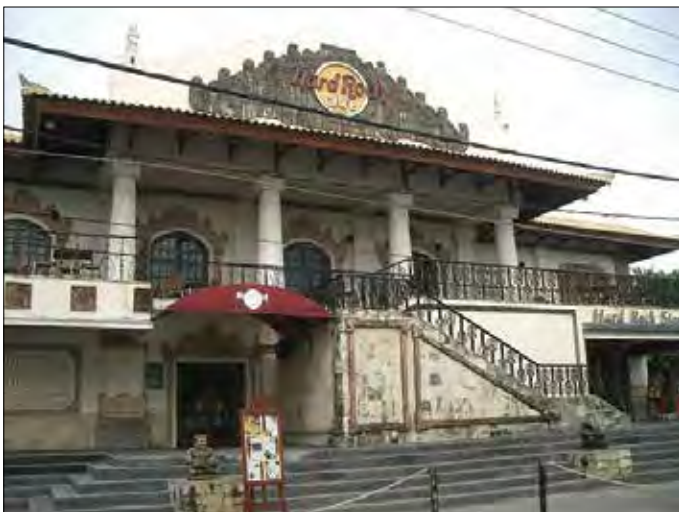
Bali (before renovation)
