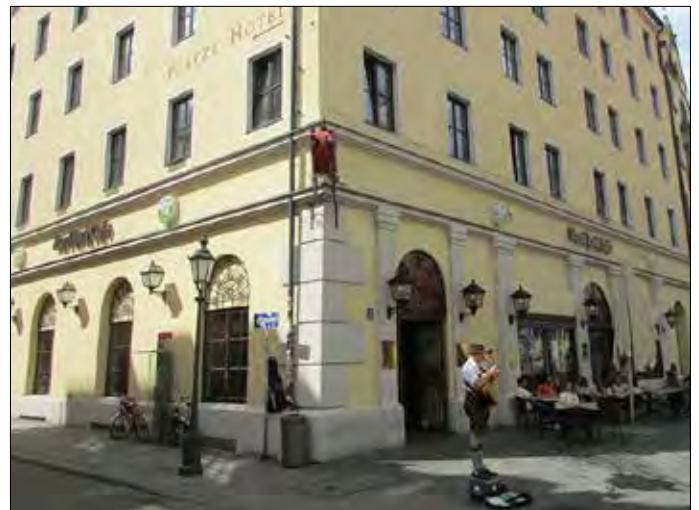
Munich (new facade)
