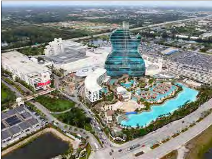
Hollywood Hotel and Casino Photo courtesy Hanson Engineering
