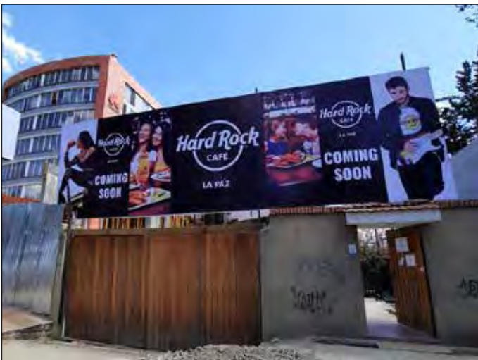
La Paz (new location under construction)
