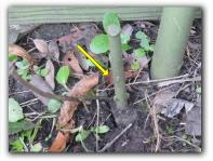
The grounding conductor was not connected to the grounding rod on the right side of the property. The purpose of this grounding rod should be evaluated by a qualifies professional.
