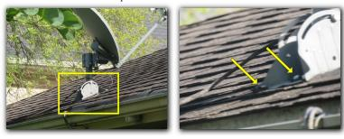
Evidence of prior repairs with sealant was observed on the roof vents. All repaired areas should be monitored on a continual basis and sealed as needed to reduce the risk of water intrusion.
