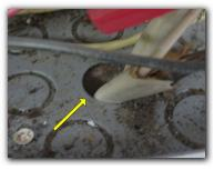
Gas pipes on the property were observed to be not bonded to the electrical system. Current electrical standards require that the gas pipes should be bonded to electrical system for safety reasons. This condition should be corrected by a qualified professional.
