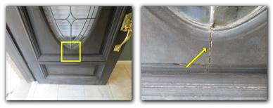
Multiple doors were observed to be out-of-square. This may be an indication of structural movement, substandard installation or door hardware issues.
