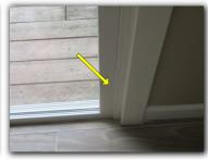
The latch bolt on the door lock is not latching in the strike plate in Backyard Door. Door hardware should be repaired and/or replaced as needed for proper operation of door and safety reasons.
