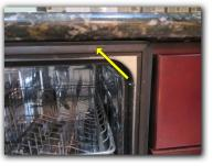
The dishwasher lacks an air gap device or a high loop. Air gaps are now standard equipment to assure a separation between supply and waste water. It is advised that one be installed or the waste pipe properly configured to prevent back flow of waste water into the dishwasher.
