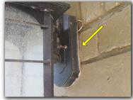
Multiple light fixtures installed on the soffit's in the exterior of the property were observed to be inoperative and/or missing the fluorescent lamps and light covers. This should be further evaluated by a qualified professional.
