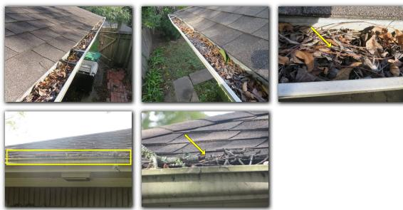
Multiple downspout's were observed to be missing. The downspout's can be installed to improve the drainage of rain water away from the property.
