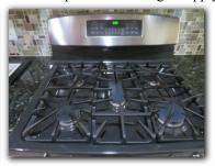
The cooking range was not secured to the wall or cabinet. An anti-tip bracket should be installed for safety reasons to avoid the cooking range from tipping over and causing injury.
