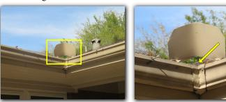
Nails were observed to be under driven on the gutter on the right side of the property. The nails should be fully driven to secure the gutter to the eave.
