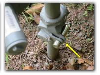
Sediment trap was observed to be not installed in the gas supply piping. The sediment trap serves as a collection chamber for sediment and moisture to reduce the risk of clogged gas valve(s) or burner(s). This should be corrected by a qualified professional for proper operation of the heating unit.
