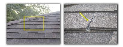
Dish mount fasteners were observed to be exposed on the roof and should be sealed to reduce risk the of water intrusion. All roof penetrations should be examined and sealed as needed.
