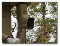
Splash blocks were observed to be missing under multiple downspouts. Splash blocks can be added to prevent soil erosion and for proper drainage of rain water. Rain water should flow away from the structure at the points of discharge, at least 3 feet away from the foundation.
