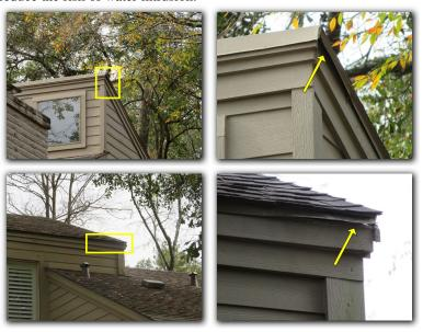
Debris was observed on the roof and can be removed to prevent future damage.
