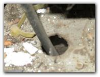
Gas and water pipes on the property were observed to be not bonded to the electrical system. Current building standards require that the gas and water pipes should be bonded to electrical system. This condition should be corrected by a qualified professional for safety reasons.
