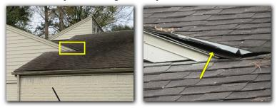
The vent flashing was observed to be loose and should be secured to reduce the risk of water intrusion.
