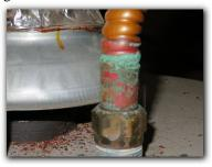
Foil was observed to be wrapped around the water heater vent flue. This is not an approved and recommended method of installation and repair.
