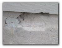
Post tension cable ends were observed to be exposed on the foundation beam. All exposed cable ends should be sealed to reduce the risk of corrosion and foundation damage.
