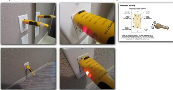
Several outlets were observed to have open ground in the Drawing Room. These outlets and the circuits should be evaluated and corrected by a qualified professional for safety reasons.
