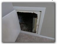
Insulation was observed to be Up to 4 inches thick on the attic floor. Current building standards recommend 13 - 14 inches insulation thickness for most southern climates. This can be improved or additional insulation can be installed as needed.
