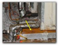
Damaged and/or missing insulation on the refrigerant line was observed at the evaporator coil unit in the attic. The cold copper tubing in contact with warm humid air causes moisture in the air to condense and then drip off of the refrigerant line. This should be repaired and/or replaced to reduce the risk of moisture intrusion.
