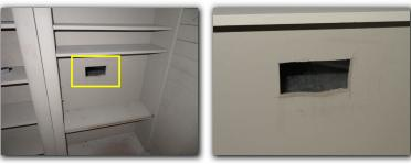
The attic access doors were observed to be not insulated. It can be weather stripped and/or insulation installed to increase the efficiency of the heating or cooling system.
