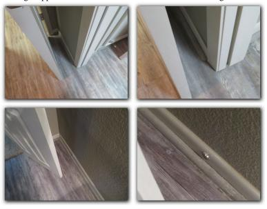
The door is not latching properly in the Master Bathroom. Door hardware can be repaired and/or replaced as needed for proper operation of the door.
