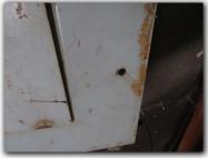
The electrical panel screws were observed to be replaced with sharp pointed sheet metal screws. These screws are unsafe and can pierce and/or damage the panel wiring. These should be replaced for safety reasons.
