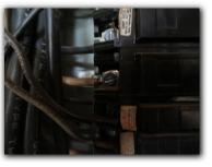
Neutral and Ground wires were observed to be double tapped under one lug. Current electrical standards require that neutral wires cannot be double tapped and a neutral and a ground wire cannot share one lug. This should be corrected for safety reasons.
