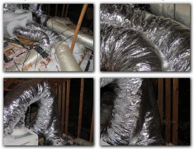
Several ducts were observed to be lying on insulation on the attic floor. Current building standards recommend that the ducts should be properly strapped above attic insulation at 4 foot intervals and hung from the rafters.
