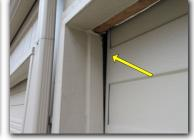
The roll-up garage door frame was observed to have a sag and separation.
