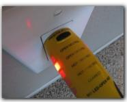
The setback in the kitchen counter receptacle outlets was observed to be inadequate. Current electrical standards require receptacle outlets installed over tile on walls or ceilings constructed of wood or other combustible materials and are set back more than 6 mm or 1/4 of an inch, the box extender's should be flush with the finished surface. All kitchen and/or bathroom outlets installed over tiles should be evaluated and corrected as needed.
