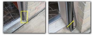
The door frame was observed to be cracked in the door frame of Front Door. This should be repaired to prevent further damage to the frame.
