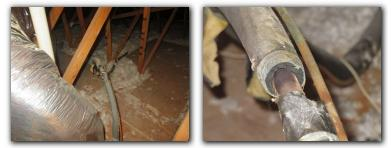
The inspector was unable to verify the visible presence of the condensate pan and drain. Current building standards require a condensate disposal assembly including pans, drains and/or a safety or float switch.
