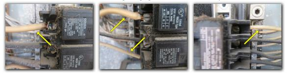
The inspector was unable to verify the visible presence and location of grounding electrode. However, all the outlets on the property were observed to be grounded when tested. Grounding wires were confirmed on the bus bar inside the main electrical panel. A licensed electrician should evaluate this inspection report and the entire electrical system for any needed repairs.
