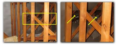
A frame brace was observed to be cracked in the attic. This should be reinforced to provide adequate strength and support to the roof framework.
