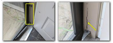
The front door was observed to be misaligned and hits/rubs the floor when opened/closed. This should be improved for proper operation of the door.
