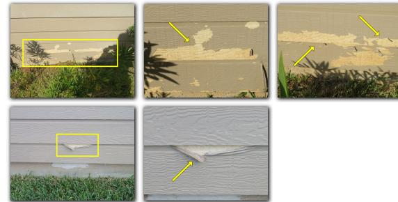
Damage was observed on the exterior siding on the back of the property and can be repaired for cosmetic reasons.
