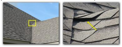
The wall flashing was observed to be loose with exposed nails on the front of the property. It should be secured and sealed to reduce the risk of water intrusion. All exposed flashing and roof penetrations should be examined and sealed as necessary.
