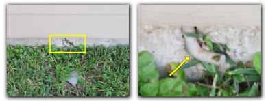
A drain pipe was observed to be exposed on the left side of the property and is not a structural concern.
