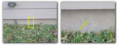
Evidence of parging was observed on the foundation perimeter beam on the right side, and, left back corner of the property. Parging is essentially a decorative mortar coat that is applied to the above grade foundation to act as a finish coat to hide surface imperfections, cracks, spalling, etc. Parging can be applied to new or existing foundation.
