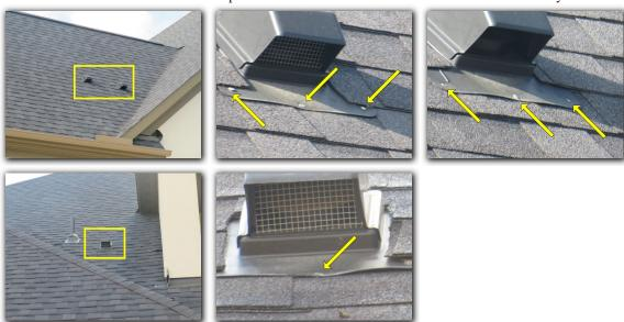
The storm collar was observed to be not seated on the base of the vent at multiple areas. This should be corrected to reduce the risk of water intrusion.
