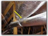
Supply air ducts were observed to be crimped between the framework and sheathing in the attic above the garage causing airflow obstruction. This should be corrected to improve the air flow.
