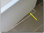
The water supply to the bath tub in the Master Bathroom was observed to be not installed and/or operational when tested. This condition should be corrected by a qualifies plumber.
