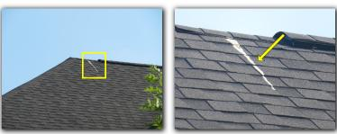
Damage was observed on the roof shingles on the front of the property. All damaged shingles should be repaired and/or replaced to reduce the risk of water intrusion.
