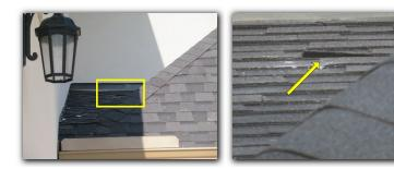
The wall flashing was observed to be loose on the left side of the property. It should be secured and sealed to reduce the risk of water intrusion. All exposed flashing and roof penetrations should be examined and sealed as necessary.
