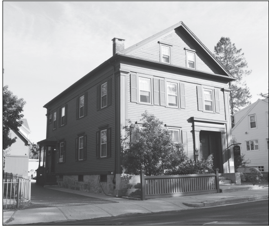
The Borden home on Second Street. Photograph, Author's collection, 2019.
