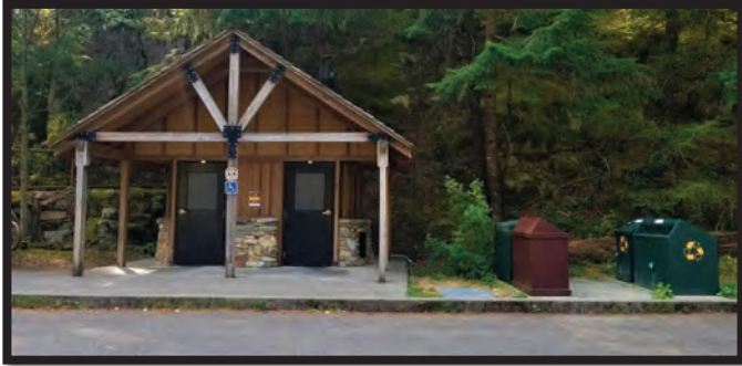
Gorge Creek Falls Parking Lot, NCNP, © 2019 J. V. L. Kiser.
