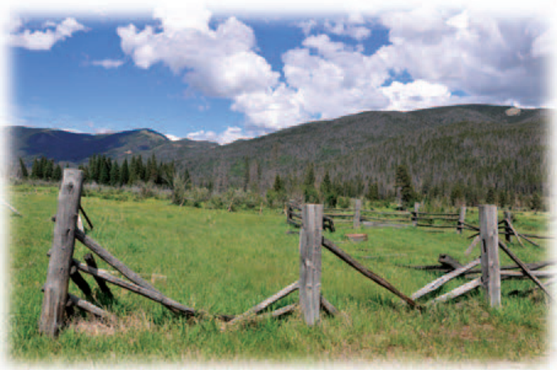
Fence Collapse at Holzwarth Historic Site, © 2015 Jonathan V. L. Kiser.
