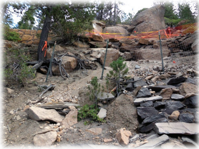
Cleetwood Cove Trail Infrastructure Repair, © 2015 Jonathan V. L. Kiser.
