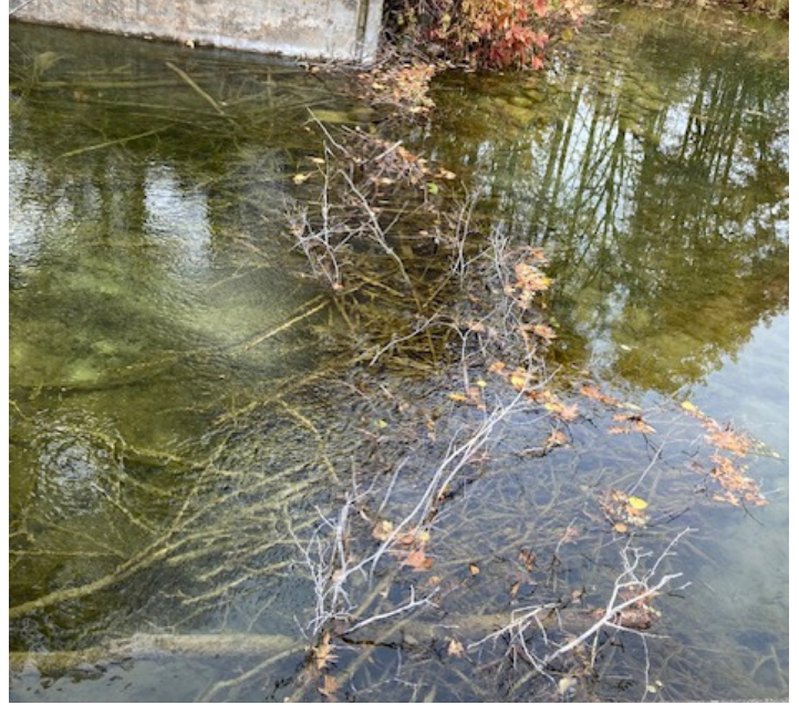
Above: Tangled brush on the weir
