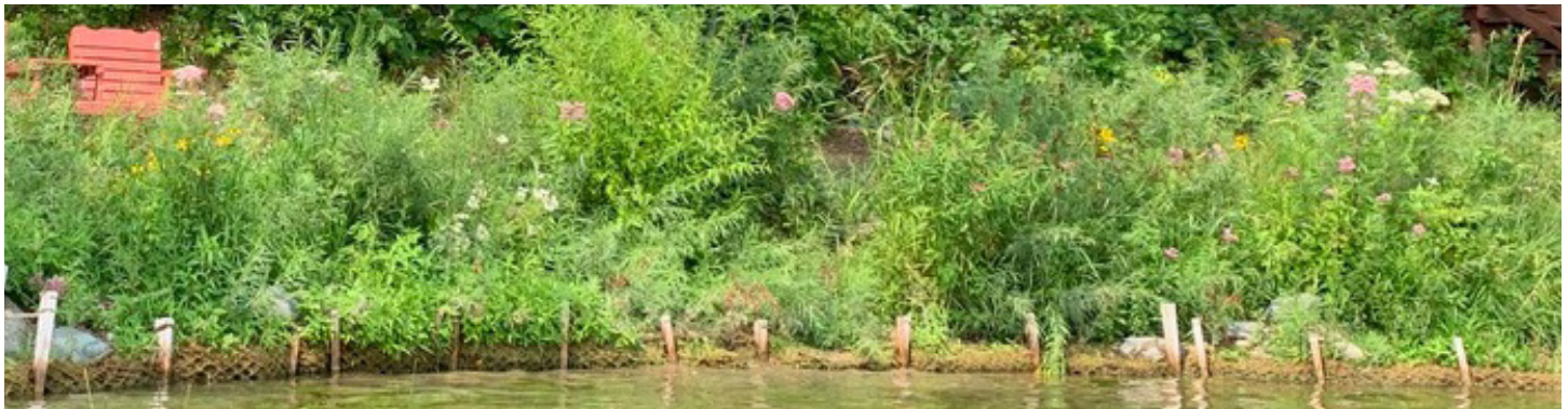
Shoreline stabilization and repair using coir logs after ice ridge damage caused erosion of the shoreline.
