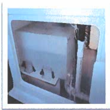
Potable Water Tank
