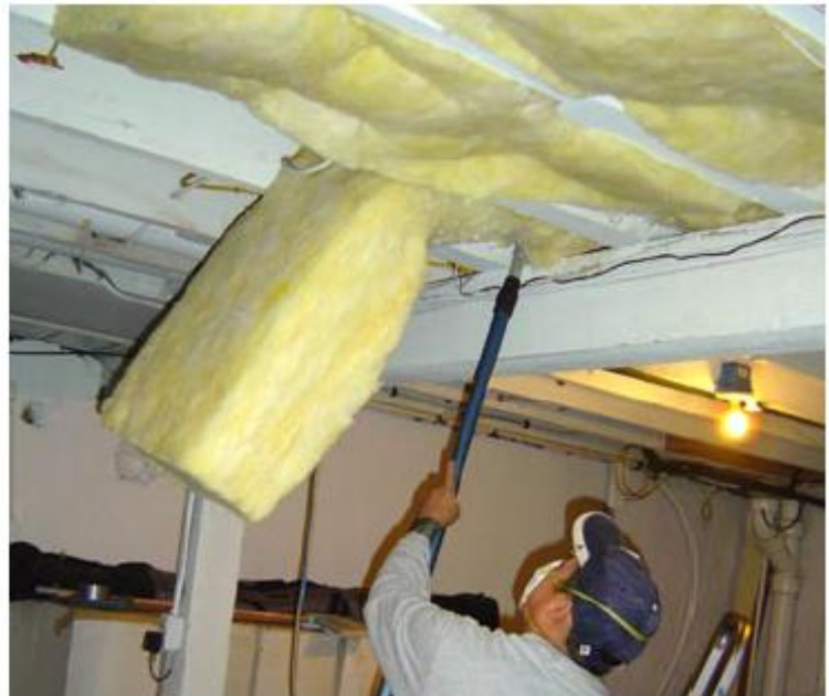
Above left: Cut fiberglass batt insulation to fit around electrical boxes, wiring and pipes that run through the walls. Compressions like the one shown above can ruin the batt's thermal alignment with the wall, which decreases its effectiveness.
