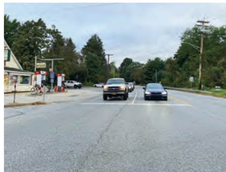
B. The street lacks sidewalks, crosswalks and bike lanes.
