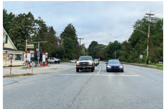
B. The street lacks sidewalks and crosswalks.
