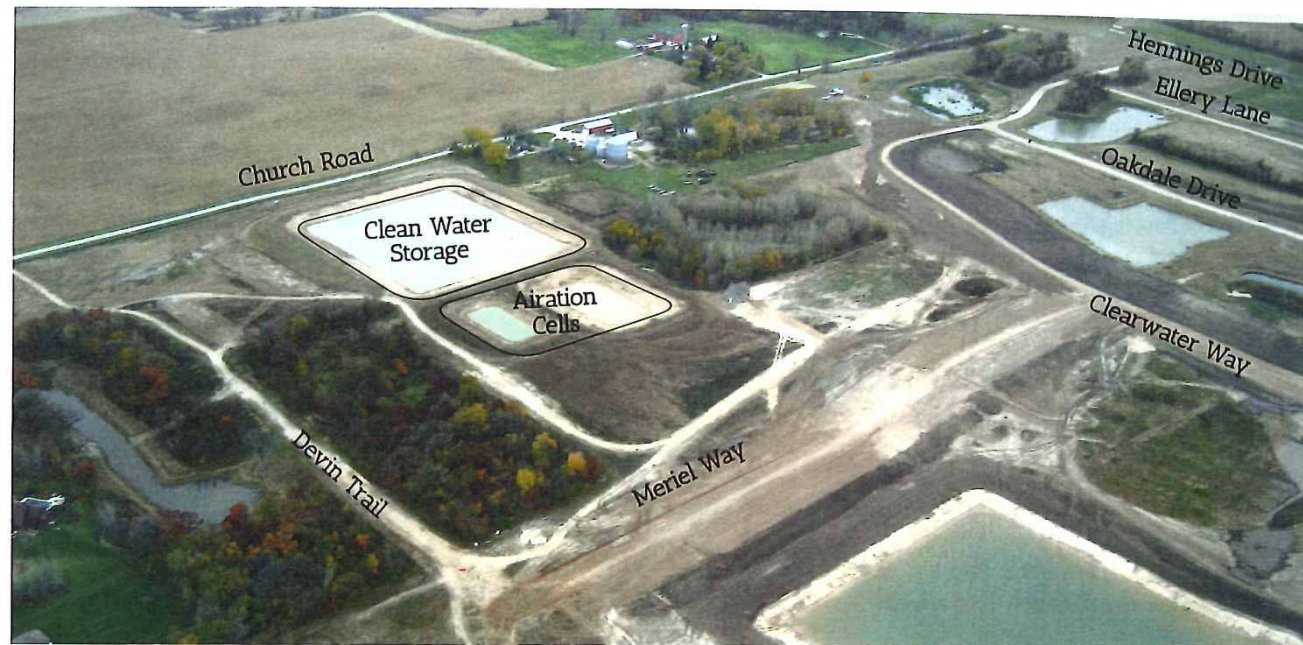
Waste Water Reclamation and Reuse System
