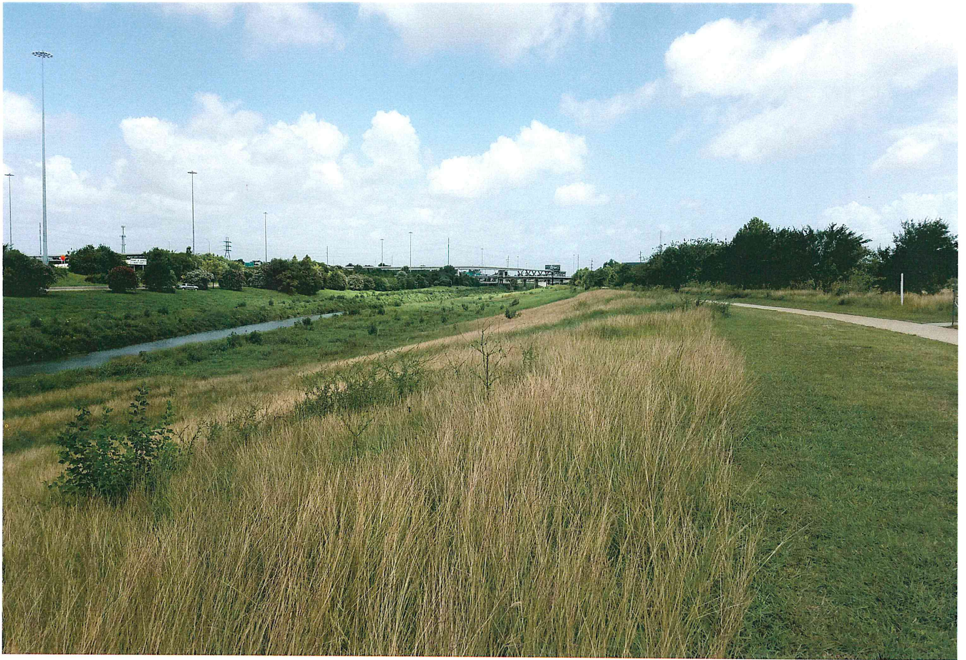
WHITE OAK BAYOU GREENWAY LOOKING NORTHWEST TOWARDS HOGAN STREET FROM THE UNIVERSITY OF HOUSTON DOWNTOWN
