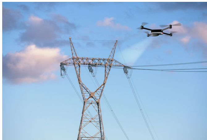
Figure 3: Utility Inspection Visualization
