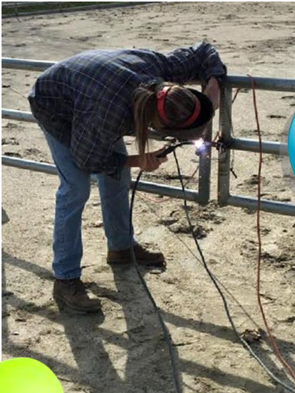
ALRC member Cary Westcott welding repair to a damaged gate latch
