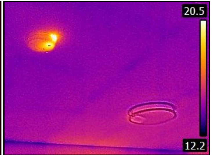
Bedroom 3 ceiling thermal scanned. No major causes of concern where visible.
