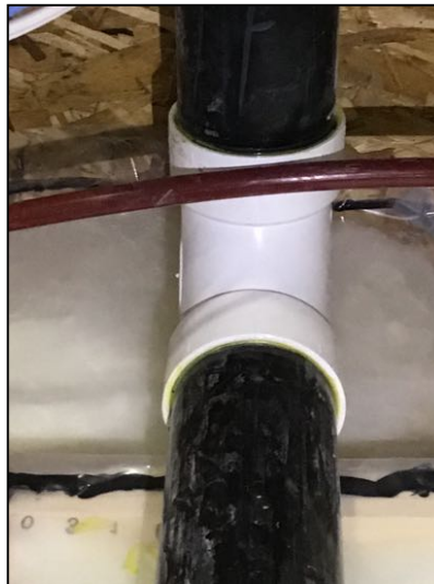
Mixture of ABS and PVC intake. ABS glue used for fittings
