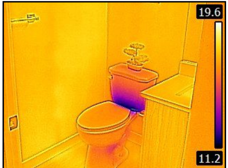
Main Bathroom - Thermal Image
