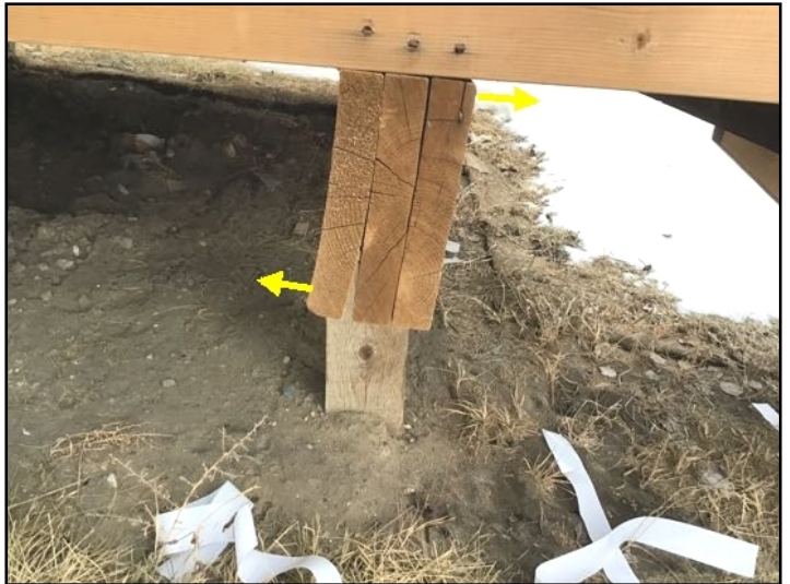
Rotating beam observed at deck. Recommend review by deck contractor
