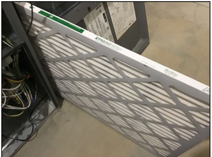
Recommend filters are changed every 2-3 months, unless otherwise stated by the filters manufacture.
