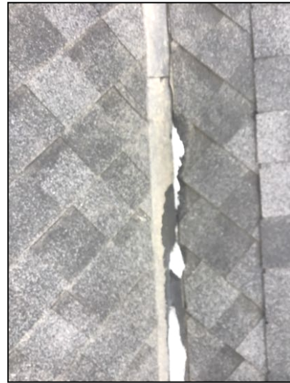
Valley flashing in serviceable condition
