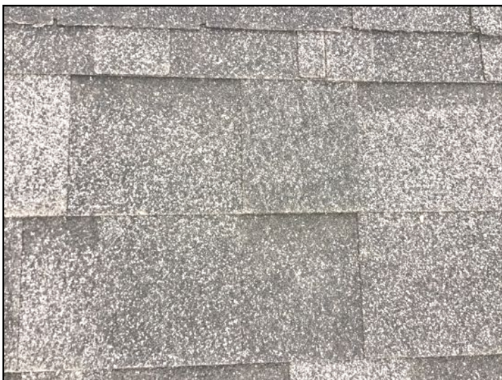
Shingles appear in serviceable condition where visible.
