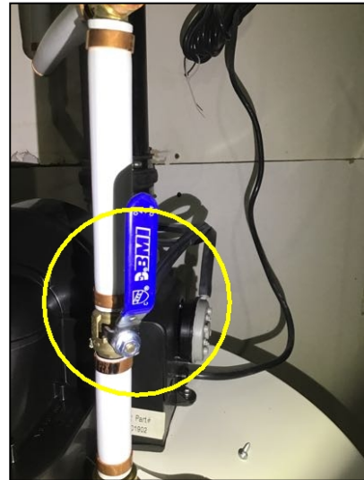
Water shut off valve
