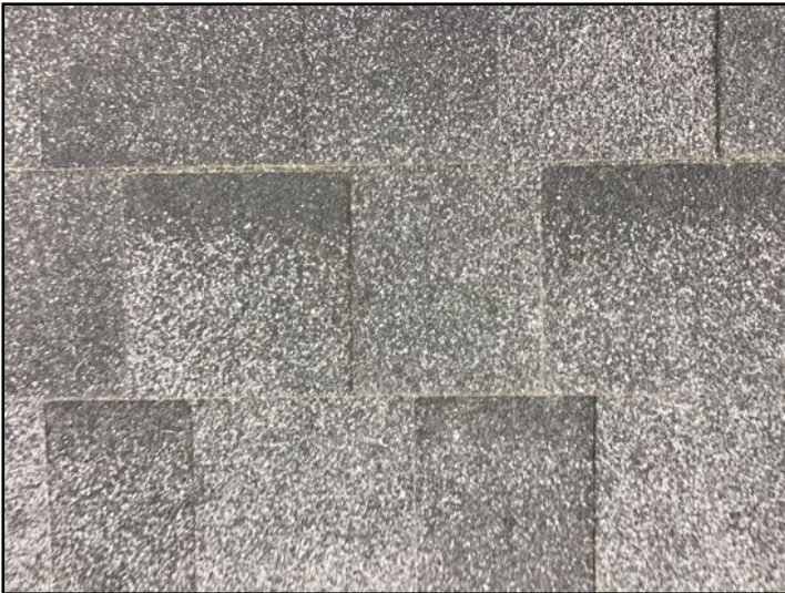
Shingles appear in serviceable condition where visible.
