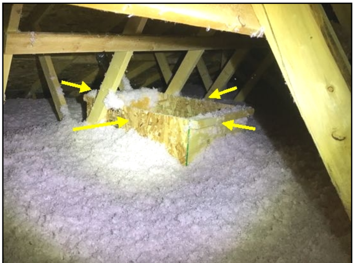
Attic hatch rough in noted. Recommend ensuring adequate insulation.
