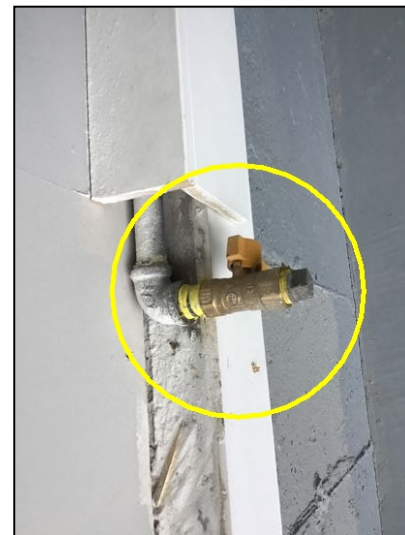
Gas shut off valve noted at garage.
