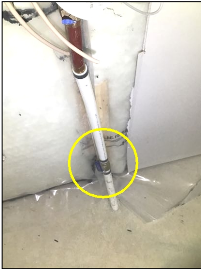
Main water shut off shown
