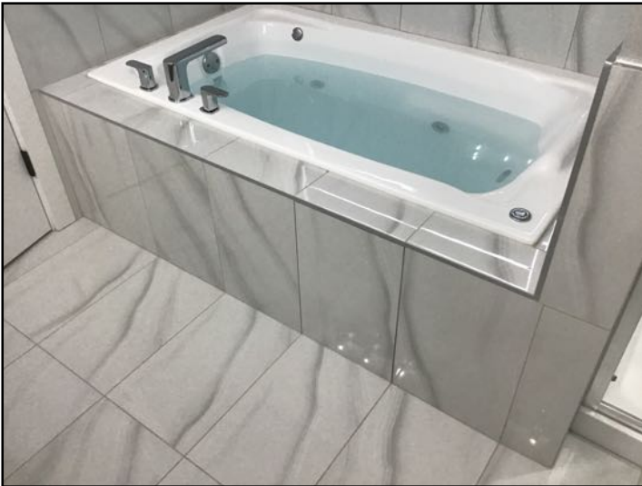
No access panel noted at whirlpool tub noted.
