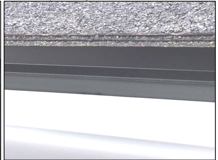
Drip edge flashing installed and appears in serviceable condition.
