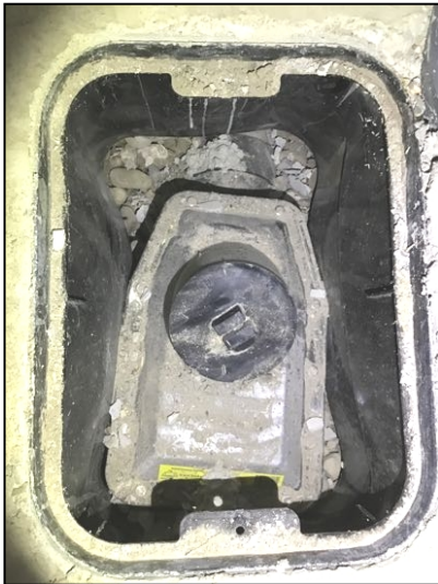
Back water prevention valve in place and appears in serviceable condition. Annual maintenance required to ensure proper operation.
