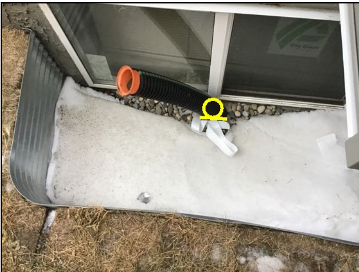
Windows observed at grade level. Wells should be cleaned regularly for proper drainage. Window well covers can be installed to keep out water, snow and debris. Recommend monitoring and grading away from window wells to prevent moisture in well.
