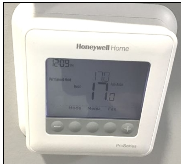
Thermostat secure on wall, and functional on day of inspection
