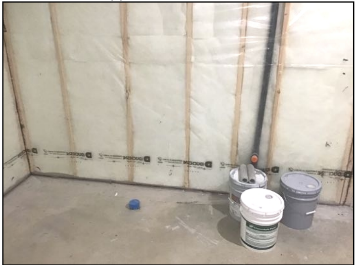
Basement Bathroom rough in
