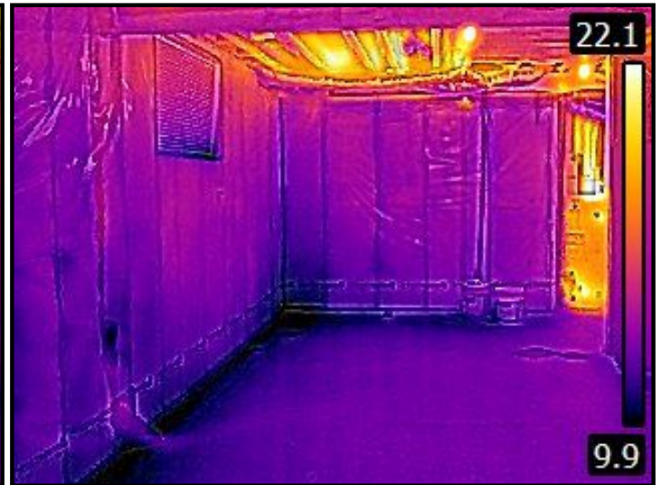
Basement dry on inspection. Insulation in place when thermal scanned
