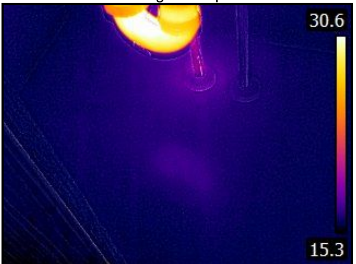
No leaks observed at the left En Suite Bathroom sink during the inspection
