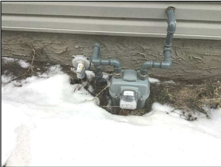
Gas meter low to ground which may affect ability to turn meter valve off. Recommend further review by ATCO for repair.
