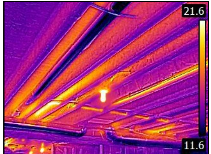
Basement ceiling dry at the time of the inspection.
