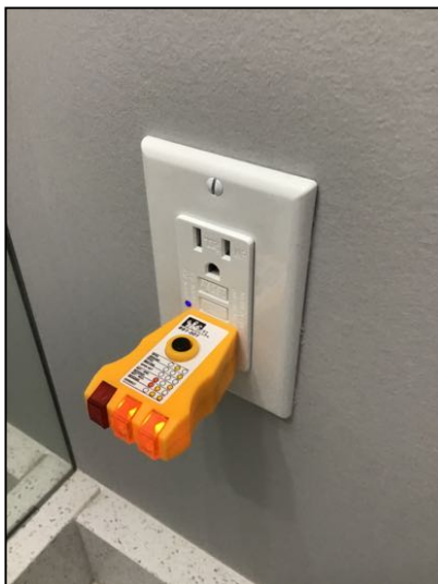
Main Bathroom GFCI did not respond to test. Suggest repair / replacement by qualified electrician for safety.
