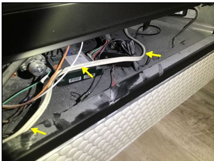
Caution: Exposed loose wiring. Recommend installing away from front access to gas control valve and remote receiver
