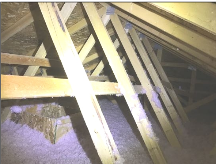
Framing appears serviceable in attic area where visible from ladders edge with flash light. Unable to determine condition of framing in areas covered by insulation or behind obstructions.
