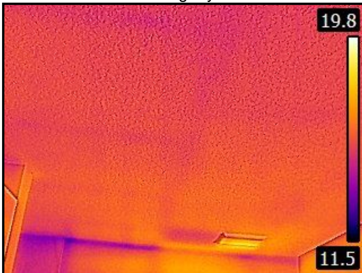
En Suite Bathroom ceiling dry on Thermal scan.
