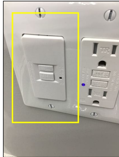
Jetted tub GFCI reset tested and working
