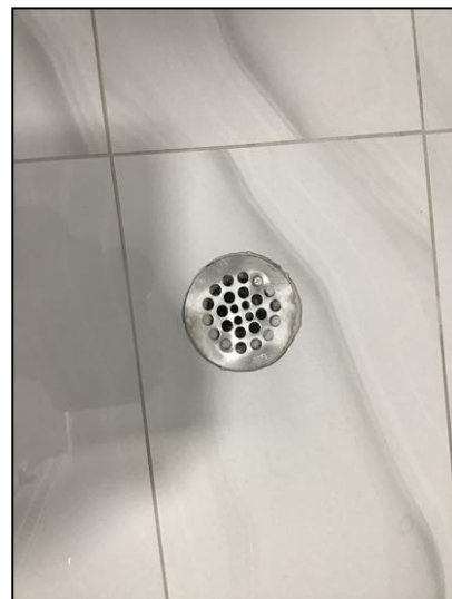
Floor drain visible.
