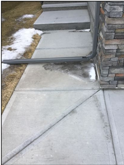
Walkway is in serviceable condition
