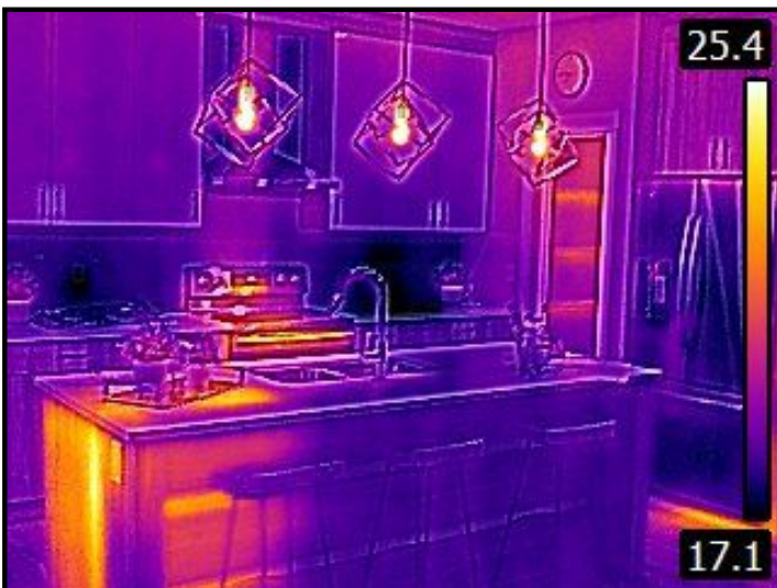
Kitchen Area - Thermal Image
