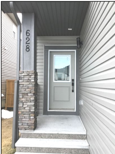
Porch is in serviceable condition.
