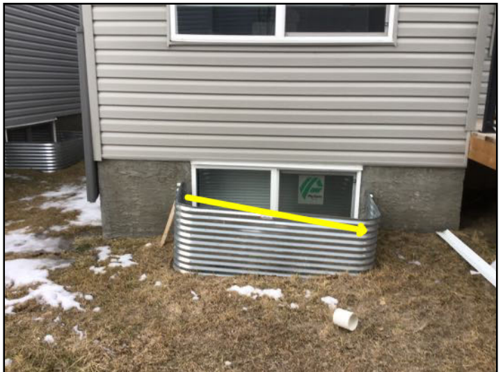
Window well has settled on right side. Recommend re-levelling.
