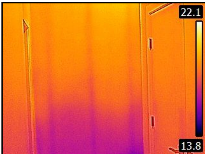
Mud Room -Thermal Image
